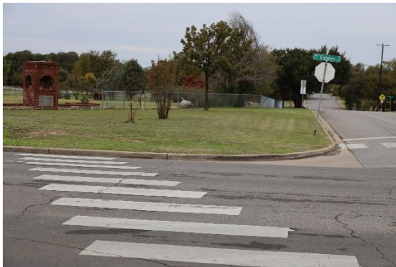
Figure 6. Pedestrian Crossing at Midway Dr with Curb Barrier and No Sidewalk
